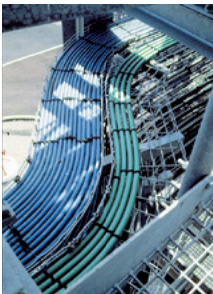
< Grouping circuits together results in a reduction of the current-carrying capacity (application of a correction factor)
