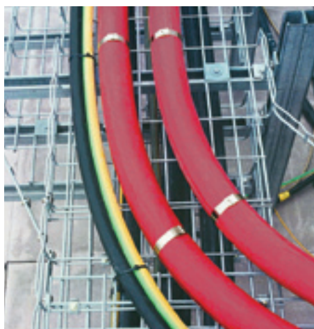
< Grouping circuits together results in a reduction of the current-carrying capacity (application of a correction factor)
